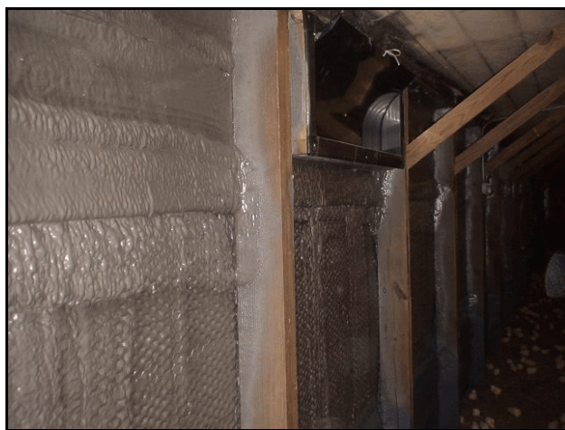
Figure 4. Side wall after polyurethane insulation was applied.
